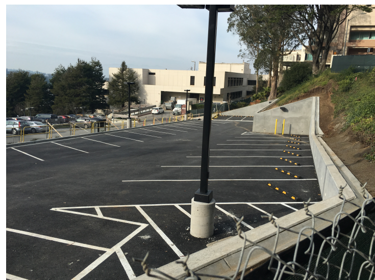
MRIV completed construction parking lot
