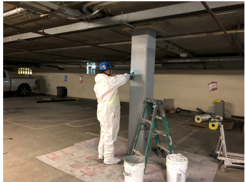
Carbon fiber wrap installed on columns in order to make stiffer.
