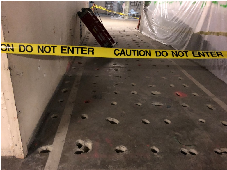
Holes drilled in the floor to accept the new metal bars.
