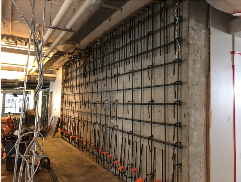
New metal bars installed in the wall to accept the new shear wall.
