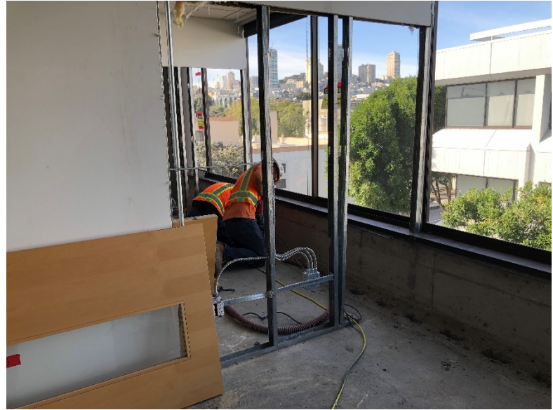
Installation of the perimeter collector beam.
