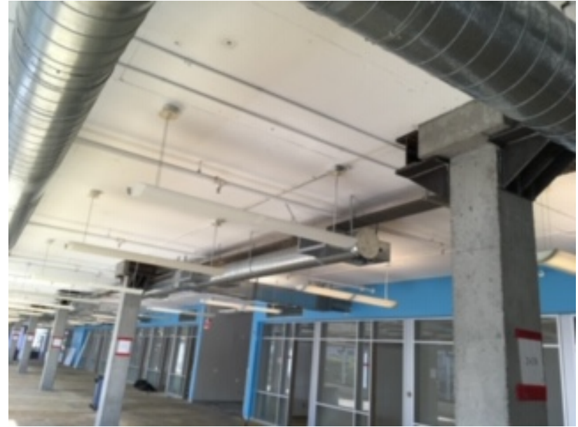
Open Office with each column capital installed.
