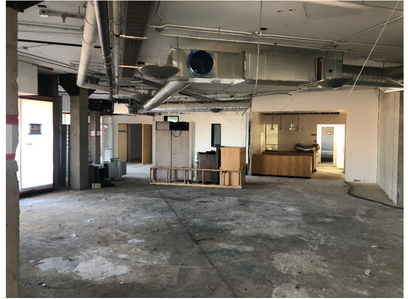
3 rd Floor Gathering Area progress.
