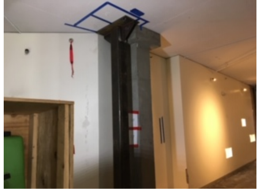
Supplemental metal column instead of column capital.
