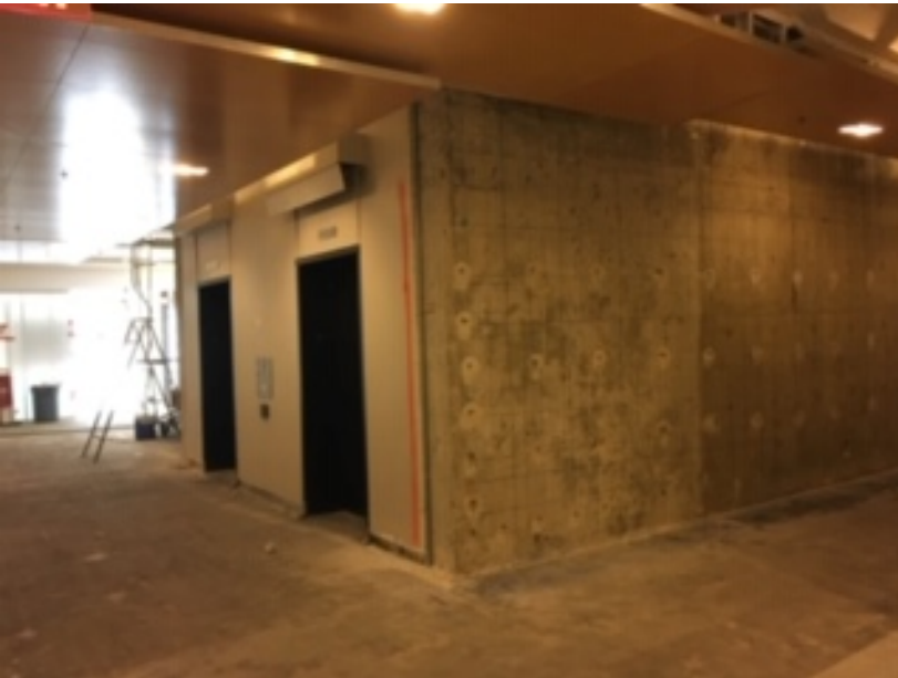
Existing shear wall prepared to accept new concrete shear wall.
