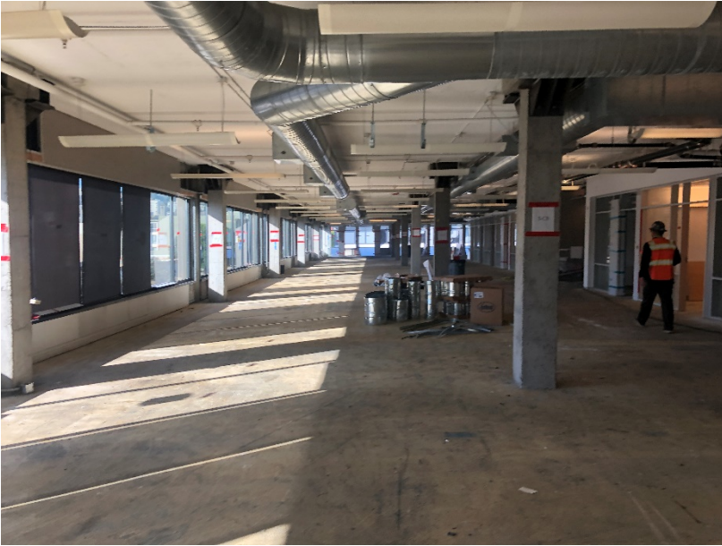
Open Office with each column capital installed.
