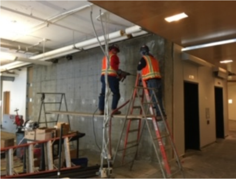
Installing dowels and rebar in existing building shear wall.
