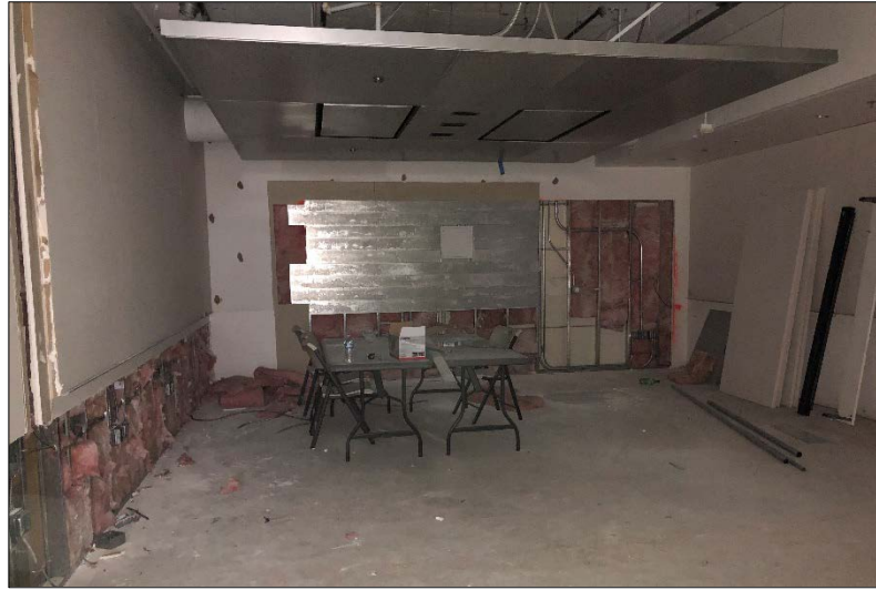
Backing and electrical/data in wall framing for new AV monitors
