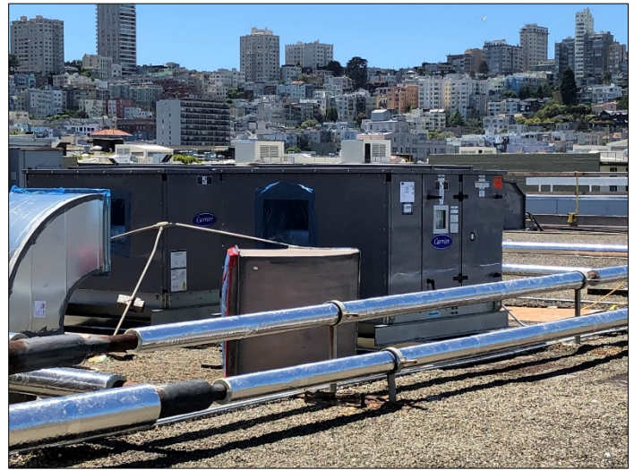
New insulation on existing pipes
