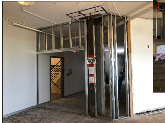
Wall framing at various locations, with electrical/data infrastructure
