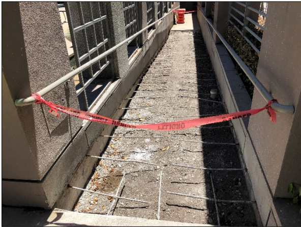
Handicap ramp improvements
