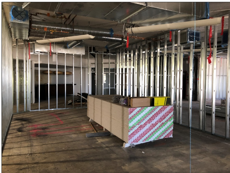
2nd Floor 202H aka Board Rm. wall framing and delivered wall board.
