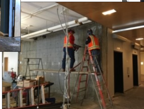
Strengthening existing walls as part of structural upgrade
